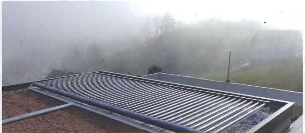
TUBO II T installation in Appenzell (CH), SPT
