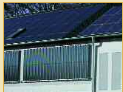
A facade mounting of TUBO 12 modules with a photovoltaic installation - Luxembourg
