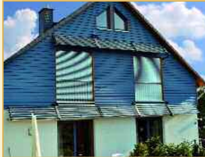
Lean-to facade mounting of 8 TUBO modules Germany
