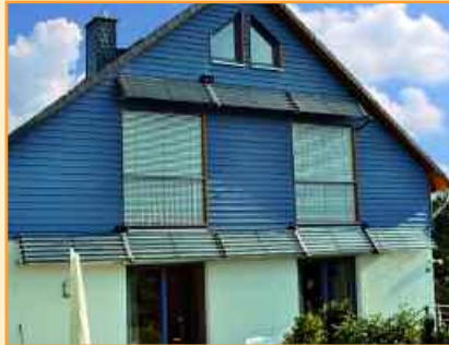
Lean-to facade mounting of 8 TUBO modules, Germany
