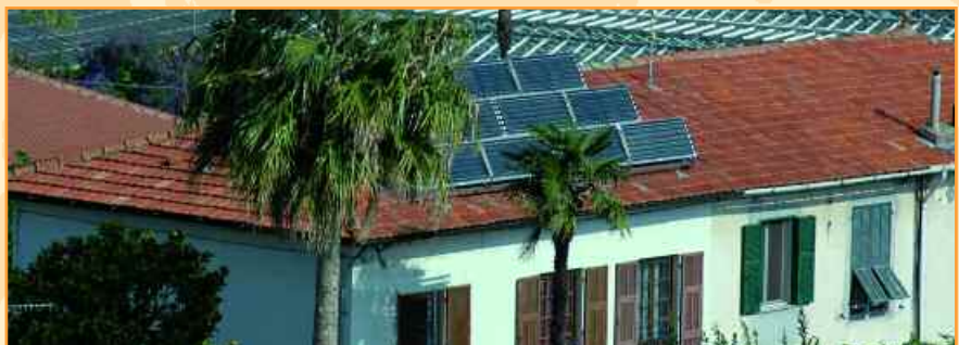
Vertically erected TUBO collectors, southern Europe
