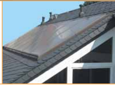
In-line roof mounted PLANO
